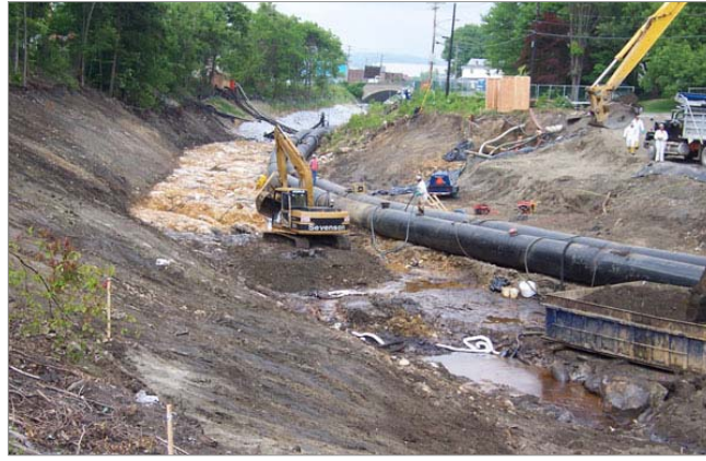
Figure 2.2: A Distressed Ecology: Dredging the Housatonic River
